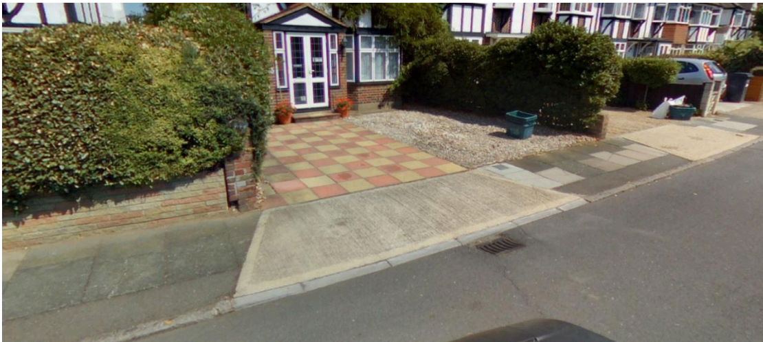
Photo 4: A Permeable Paving Hard Standing
