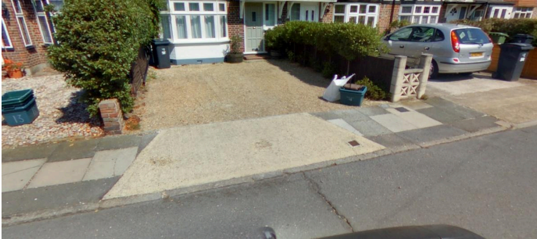
Photo 3: A Shingle (Loose Surface) Hard Standing
