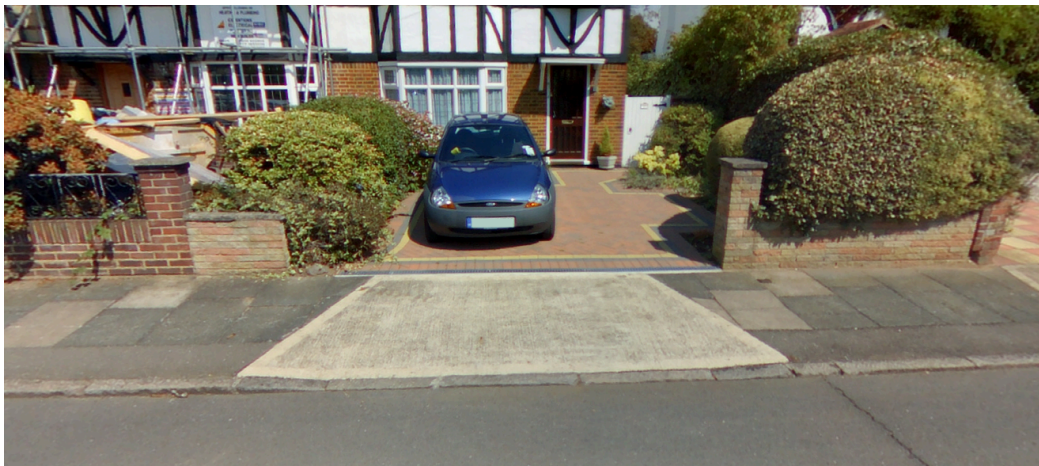
Photo 1: Typical Concrete Vehicle Crossover
